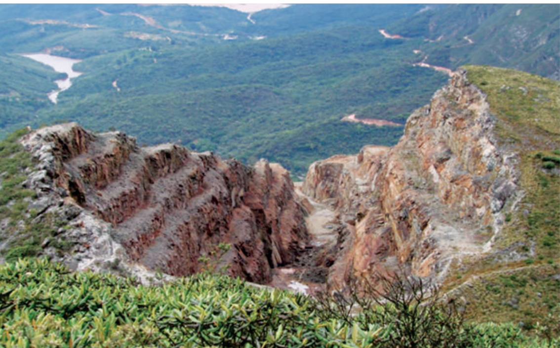
Figure 1: João Belo mine, in Jacobina. Water supply dam for the project and Yamana Gold tailings dam, respectively. (AMILTON, 2010)
